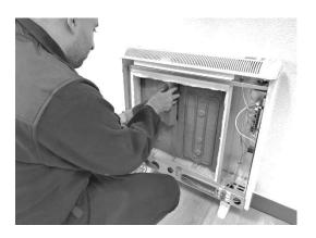
10. Place the heating elements back into their original position. Place the other two rows of storage bricks with the flat side facing out and always on the heating elements supporting tabs.
